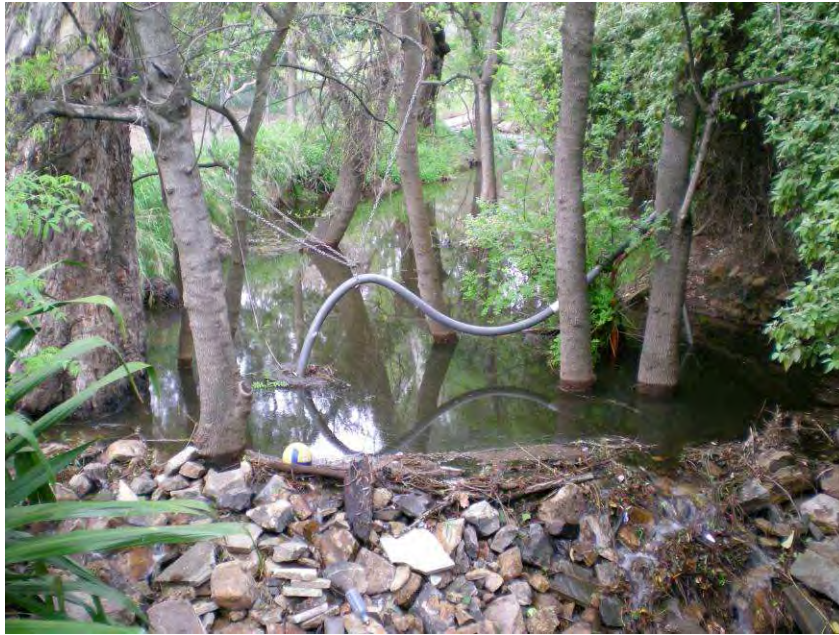
“Water being taken from Brown Hill Creek as part of local Aquifer Storage & Recharge Program” (ASR)
